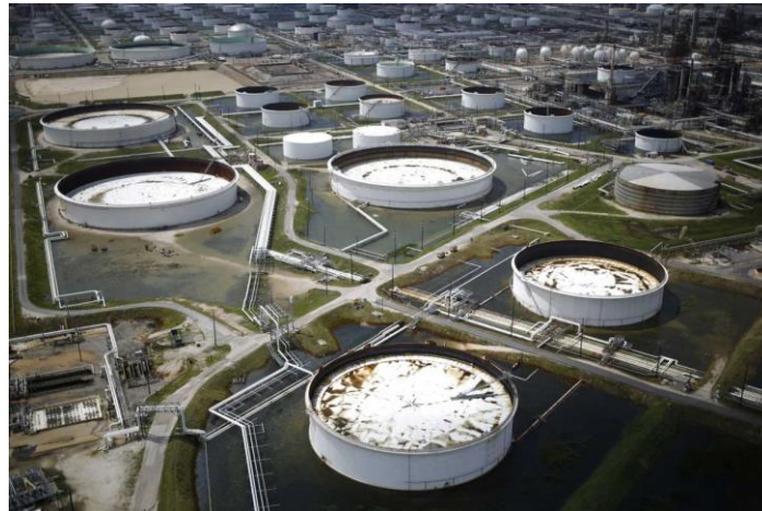
Figure 3. A View of Damaged Refineries
